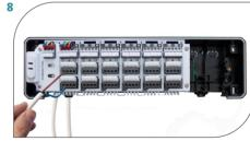
Connect the thermoelectric actuators wires.
